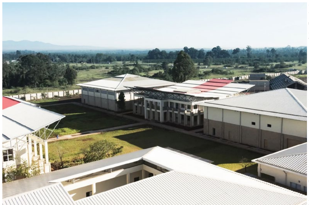
Mpresa Foundation Auditorium (center), one of the venues of the Festival
